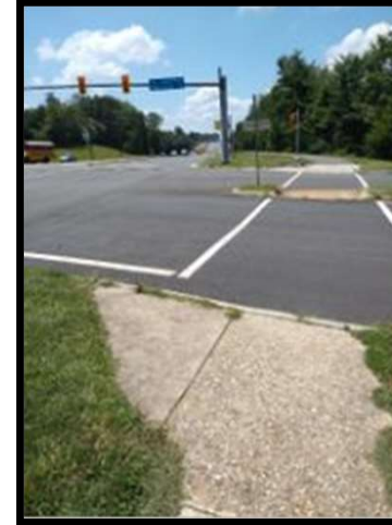
Route 29 at Ridge Top Rd
