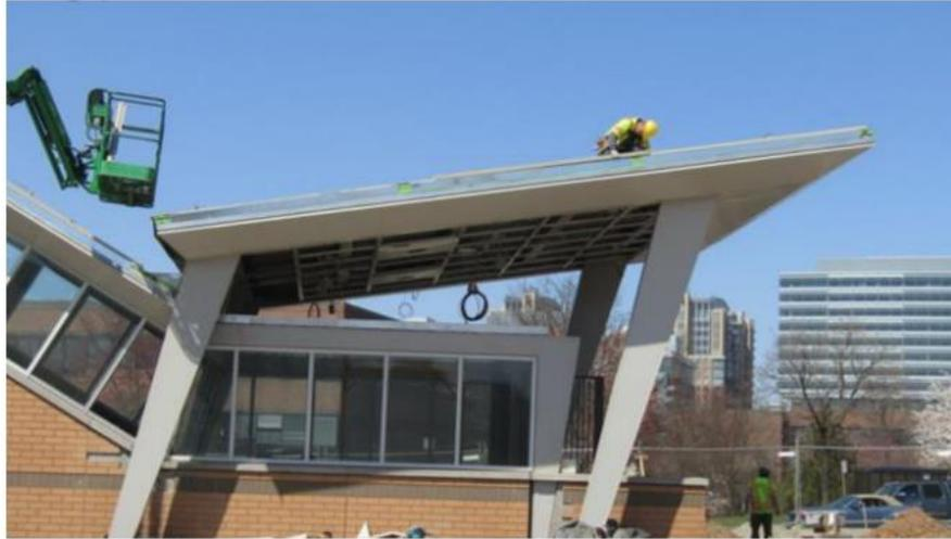
Finishing Trim Installation on the Reston Station Vault Roof
