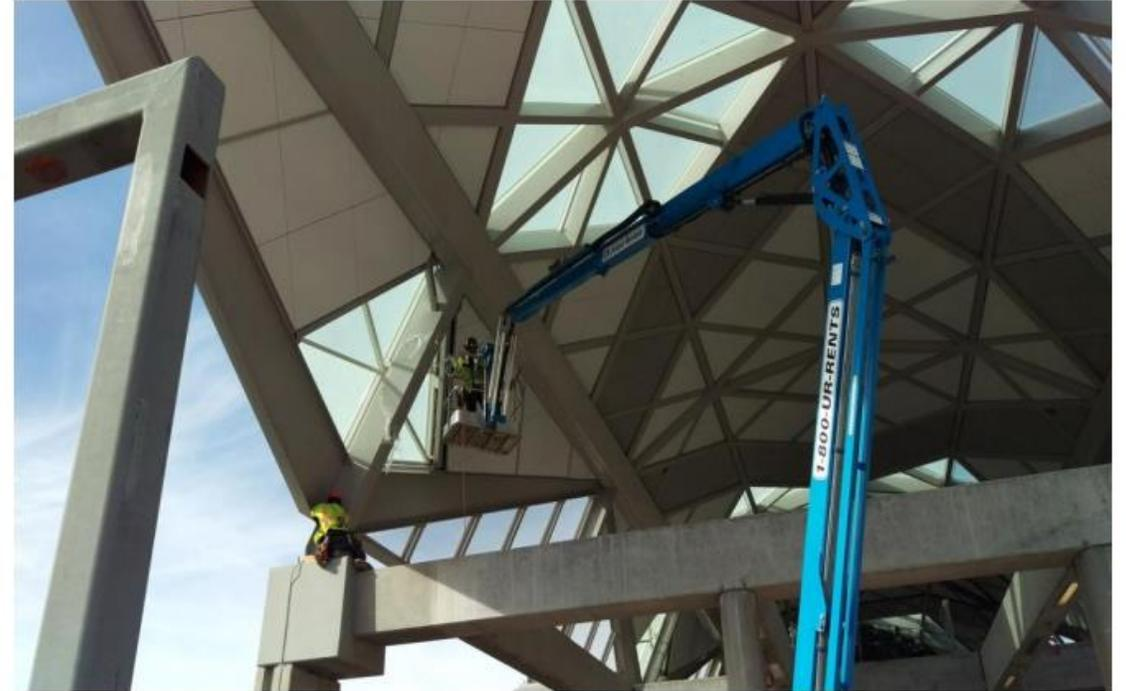
Hydro Prepping Handrail for Coating at Reston Station
