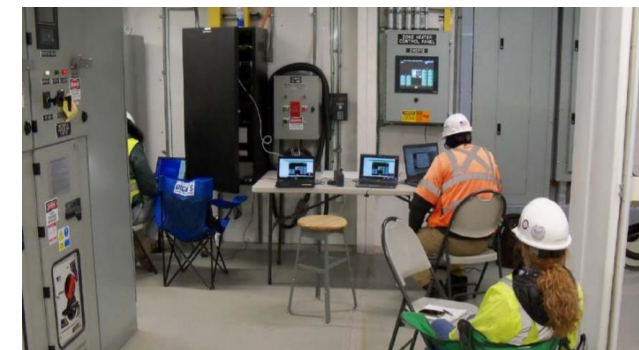
Reston Town Center Station testing
