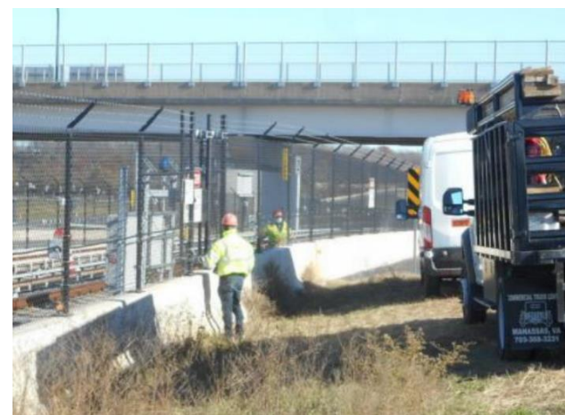
Minor Repairs to Track Walls Along Eastbound Dulles Airport Access Road
