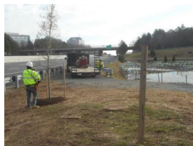
Landscaping Work along Eastbound Toll Road
