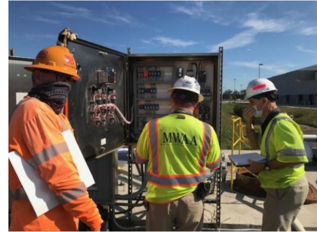
Sanitation Lift Inspection at the Yard
