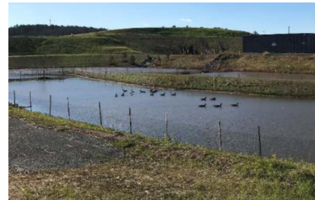
Stormwater Management Pond near Rt. 28
