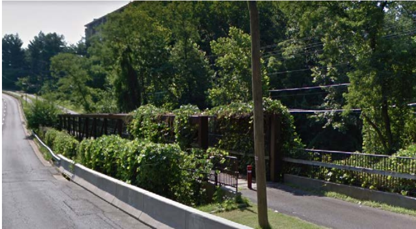
Figure 9: Existing Pedestrian Bridge by Barcroft Dam
