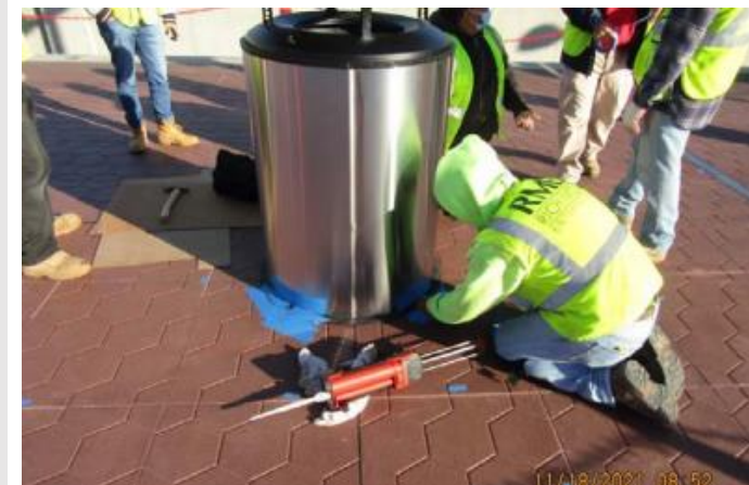
Trash Can Installation
