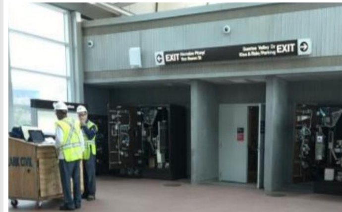
Fare Card Machine Installation
