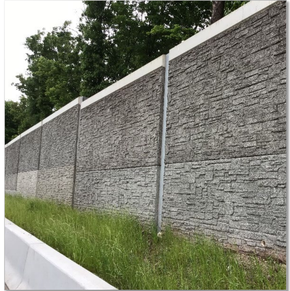
Example of dry stack (simulated stone) noise wall
