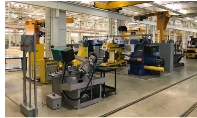
Safety and Inspection Building Outfitting
