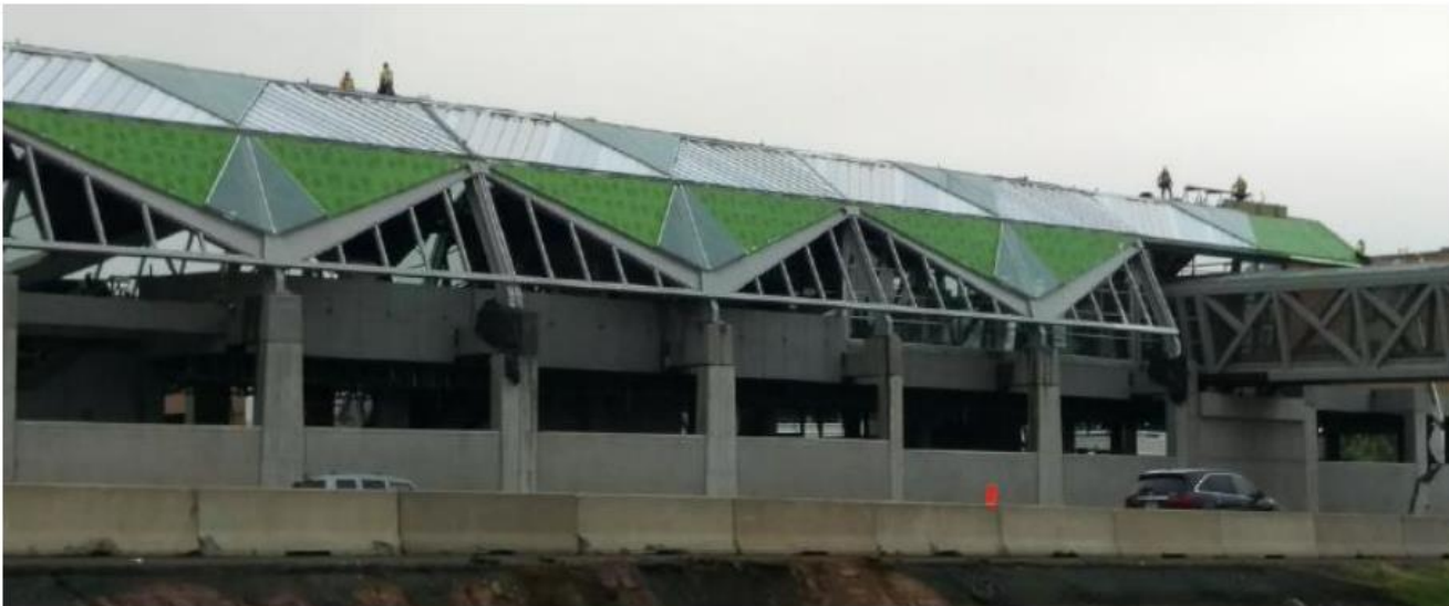
Installation of Standing Seam Roofing on Reston Station Vault Roof
