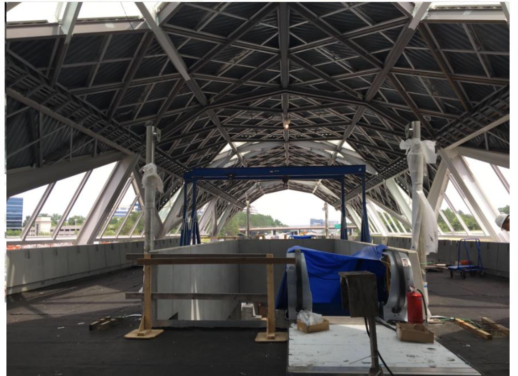
Canopy Ceiling Framing in Reston Station Mezzanine
