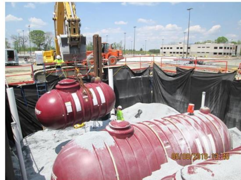
Installing Underground Storage Tanks (Gasoline, Diesel)
