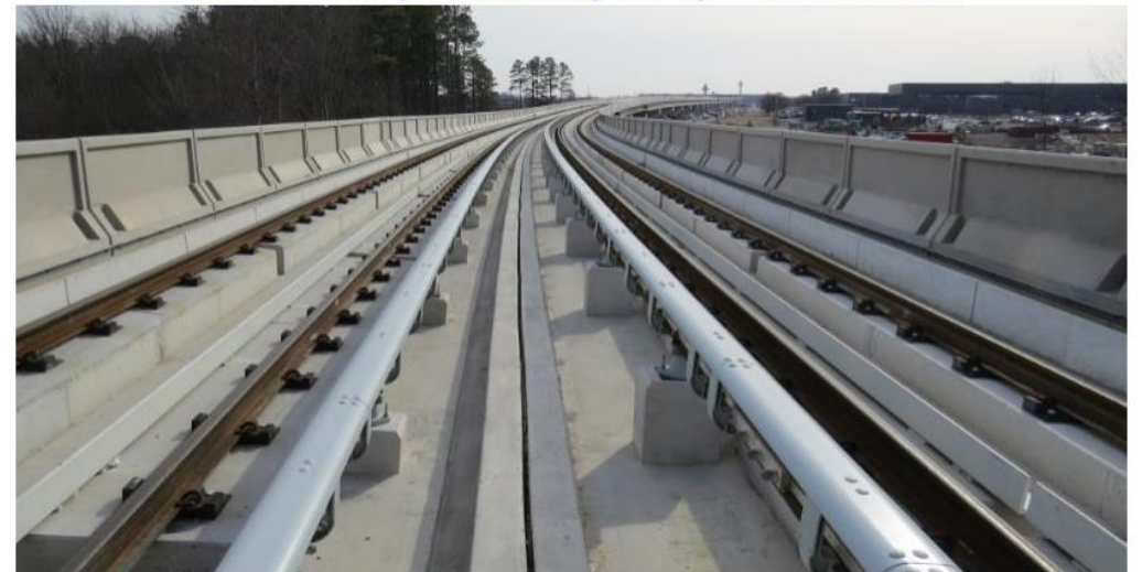
Aerial Guideway Track Ready For Systems Installation
