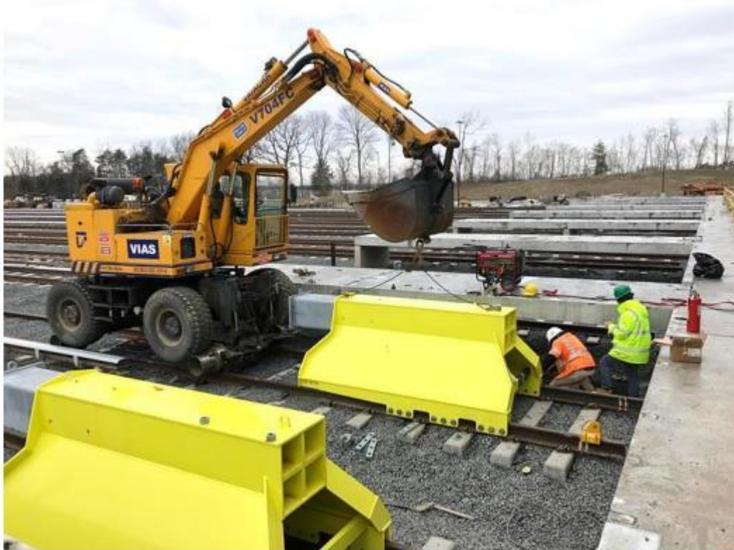
Installing Bumping Posts at the TB
