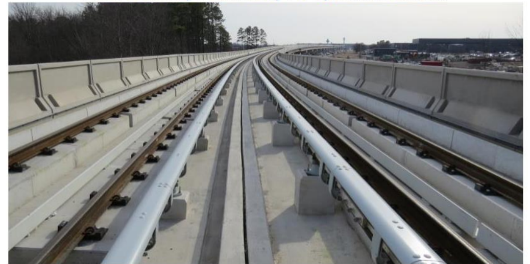
Aerial Guideway Track Ready For Systems Installation
