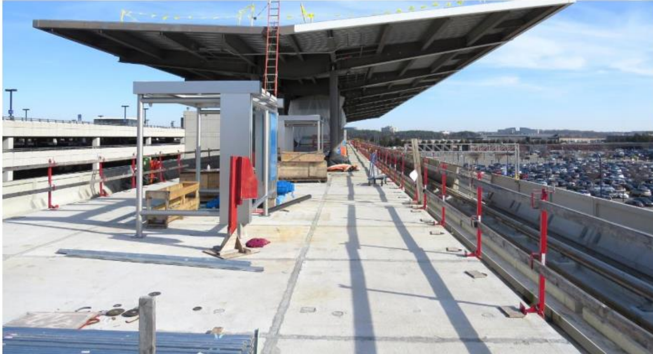
Dulles Station Platform, Canopy Roof and Guideway
