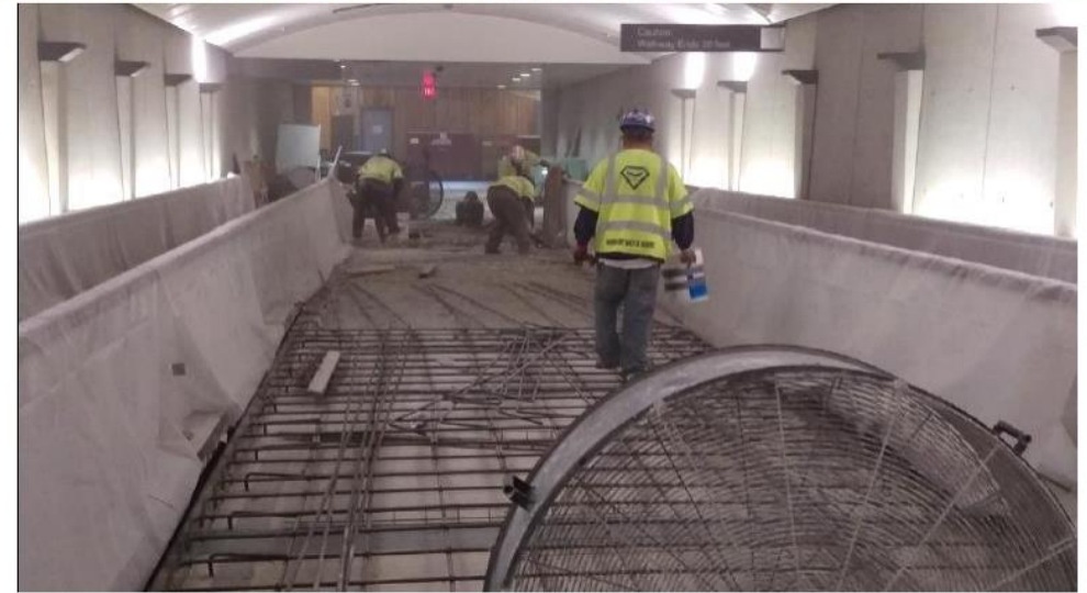
Prepare for Concrete Pour of Walkway in Pedestrian Tunnel at Dulles Station
