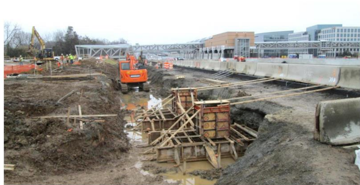
Excavate and Form Innovation North Sound Wall Foundations
