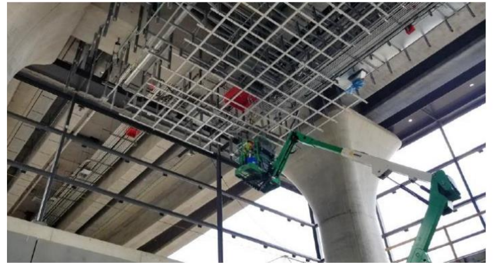
Installing Ceiling Grid in Dulles Station Mezzanine
