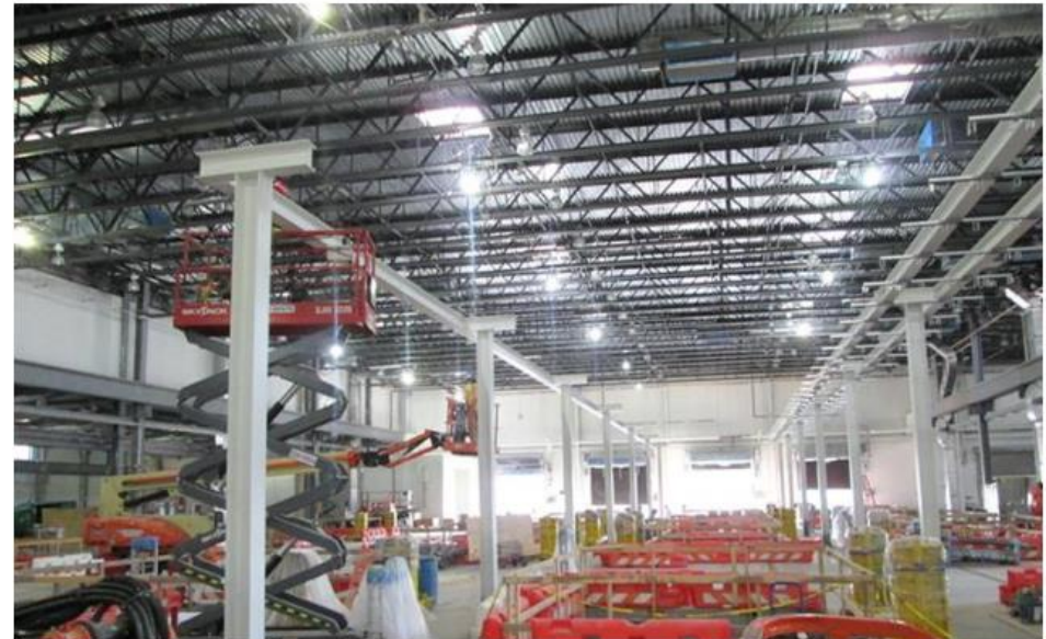
Erecting Steel Support Frame for the Stinger System in the SIB
