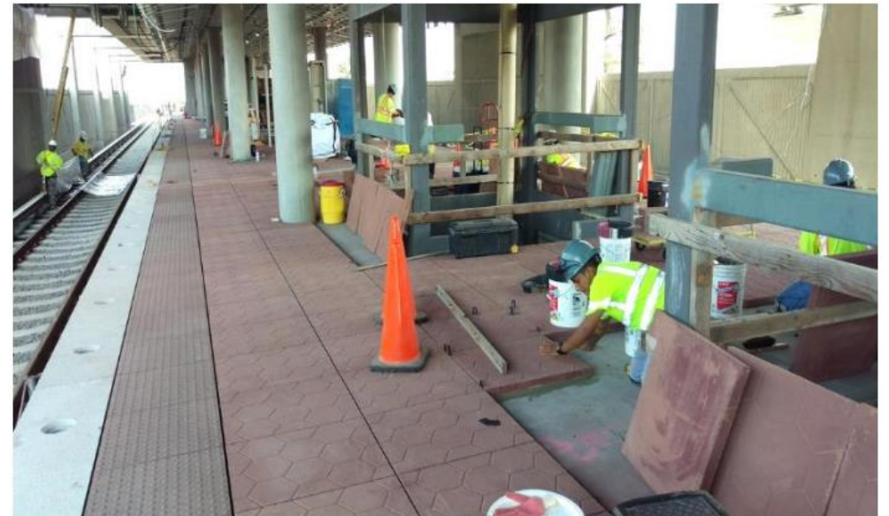
Reston Station Platform Paver Installation
