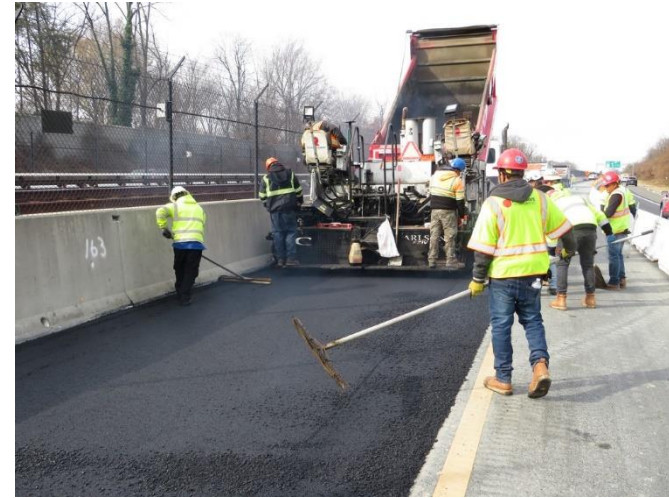
Road crew for DCR shoulder work
