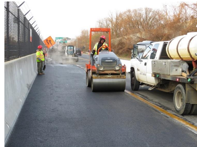
Asphalt roller on DCR shoulder
