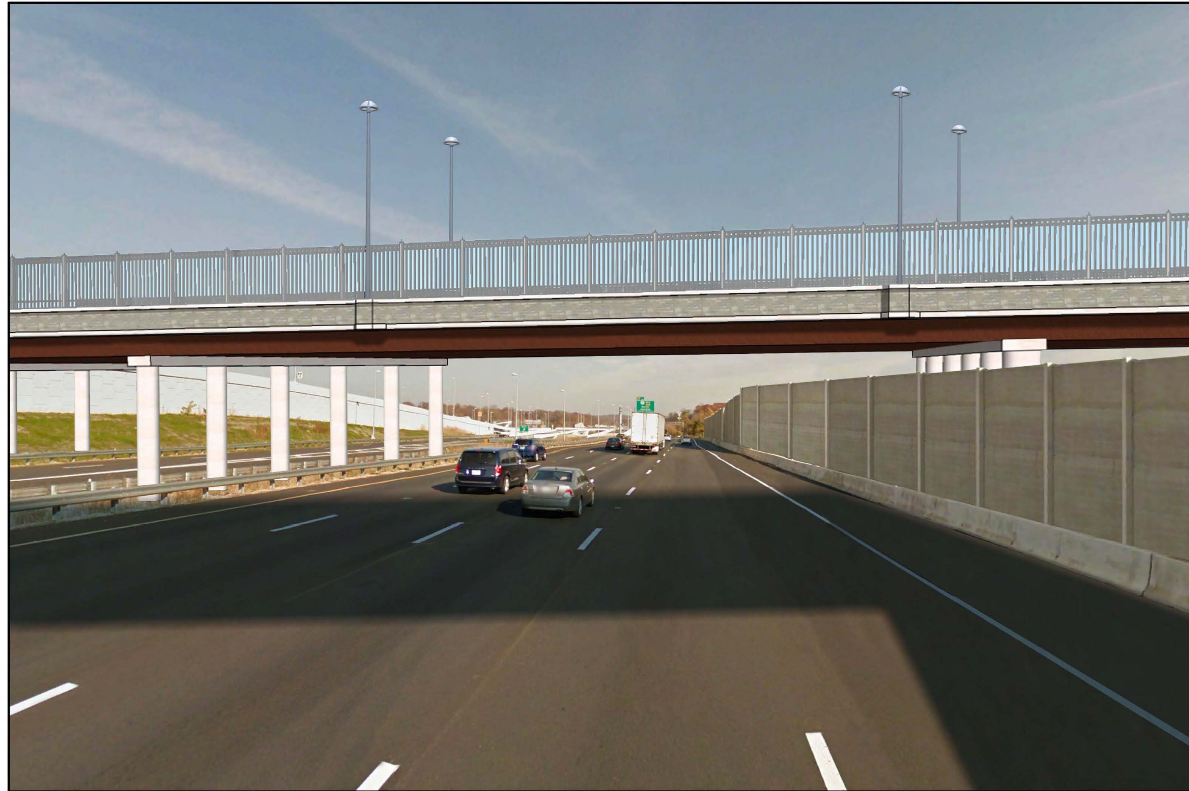
JONES BRANCH CONNECTOR BRIDGE OVER I-495 (LOOKING NORTH)
