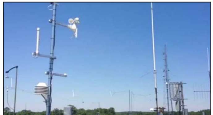
Weather station at the Virginia Emergency Operations Center. Photo by the Virginia Department of Emergency Management
